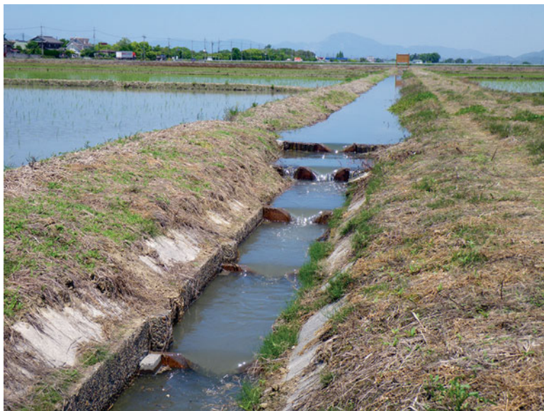
Fig. 2 A fish-ladder cascade set in a drainage canal (© Shigefumi Kanao)
