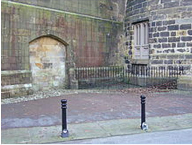
Illustration 5.1 Hanging Corner at Lancaster Castle (photographic image, supplied by the author, 2013). Note: Just outside Lancaster Prison was used as a site of execution for capital offences post-1800 until the Drop Room was opened in 1865. There was originally a drain for all the detritus at the Hanging Corner, now filled in.
